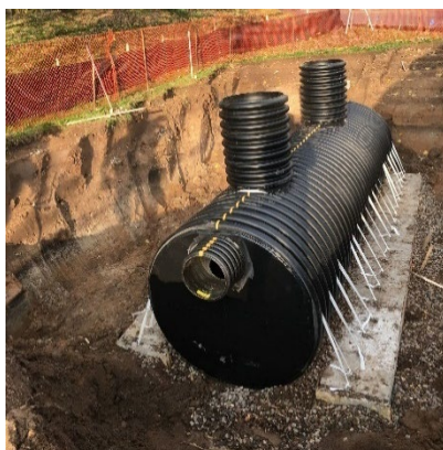
Water quality unit installation (October 2017) and Southwest Treatment Wetland (August 2018)
