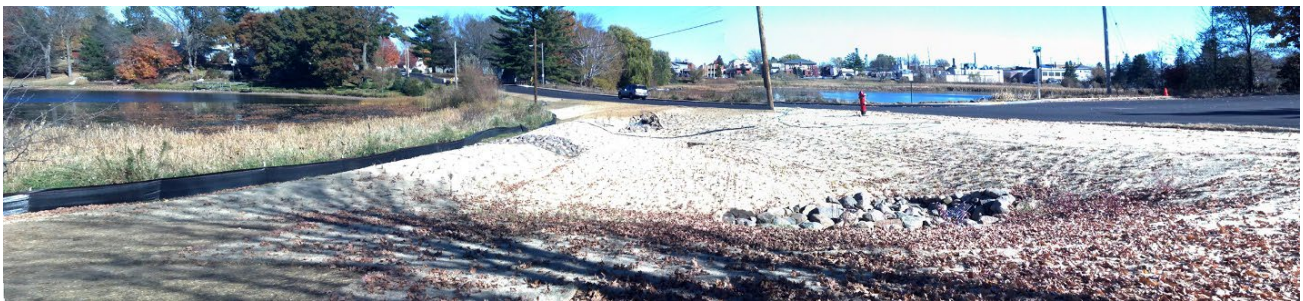
Neurer Treatment Pond October 12, 2012, right after construction
